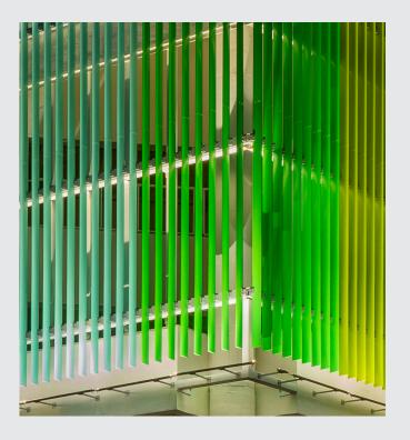
In addition to providing a unique aesthetic, CS' airfoil blades block car headlights from exiting the garage as light pollution and allow for airflow, which is important for a garage filled with cars and emissions.
