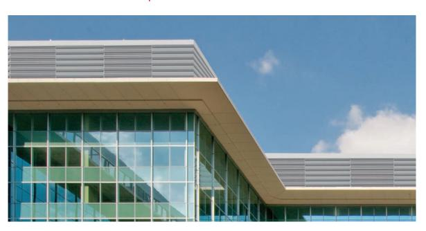
Bold Line Louvers and matching Super-Rib Panels are engineered for seamless integration. The active louver area and rainscreen wall panels share the same profile, providing a continuous run of uninterrupted bold articulations and shadows. The panels may also be insulated to add a level of thermal protection.
