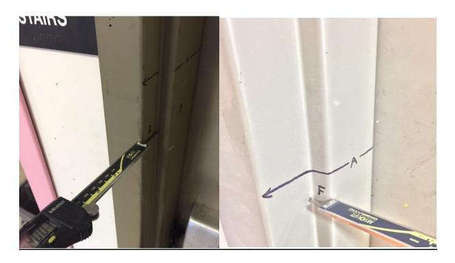
The last picture is of the "G" dimension back to the finished drywall.
