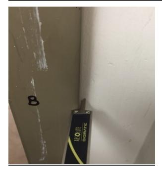
Please note: Each door frame should be measured individually to verify that there are no dimensional differences from door frame to door frame.
